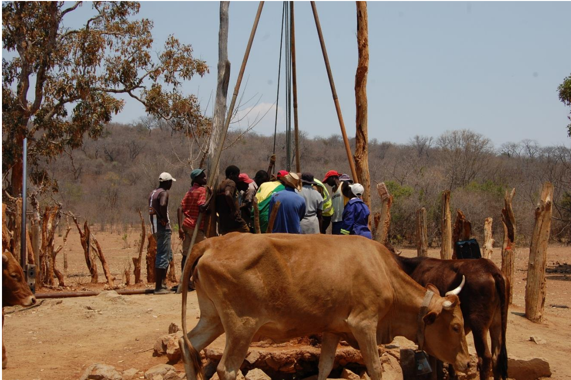
Pump minders repairing the Chigusu borehole
